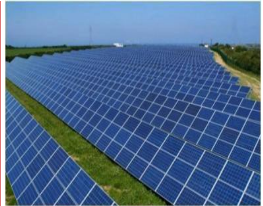
274 MW project in Ontario, Canada
